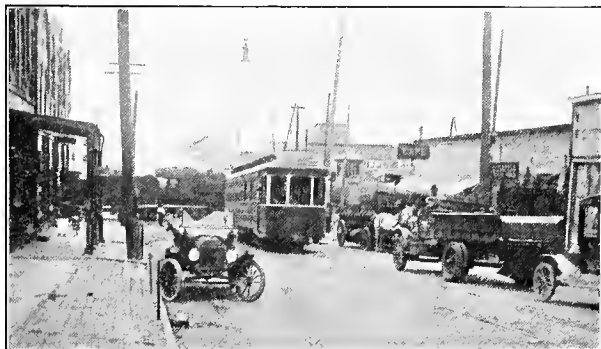
Congestion of East Exchange Street, to be relieved by grade elimination
